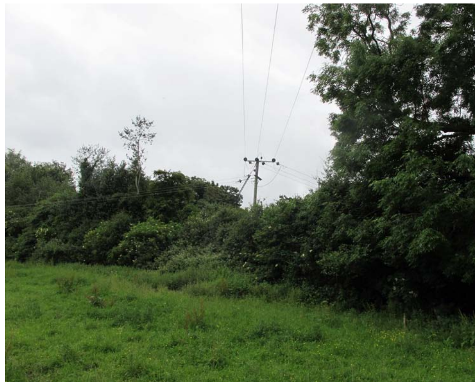
08- Overhead Telephone Lines
